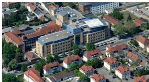
► The Johanniter hospital in Stendal from above
